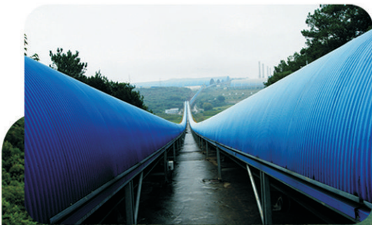
CR Cement Project, 48km double line conveyor - designed by RBLREI France
